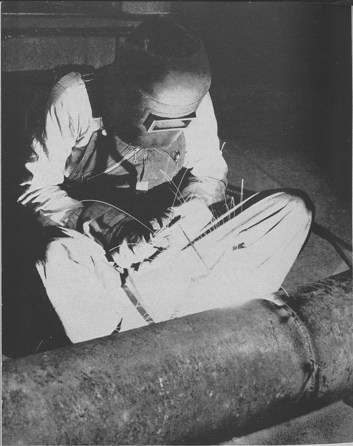
POSITION ARC WELDING ON PIPE
