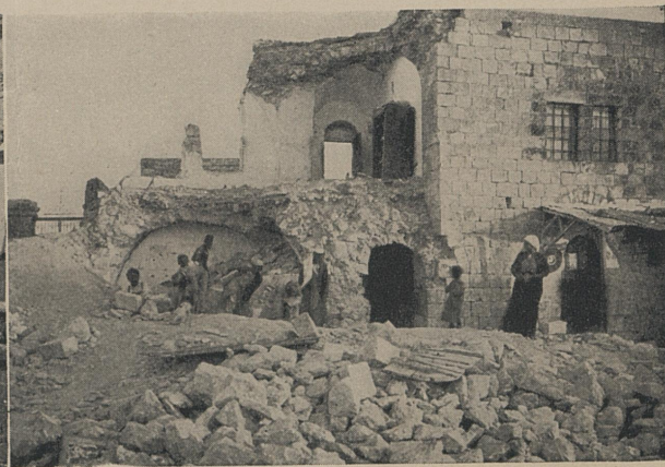
Am. Col. Photo Collapsed house, Mt. of Olives, three persons killed.
