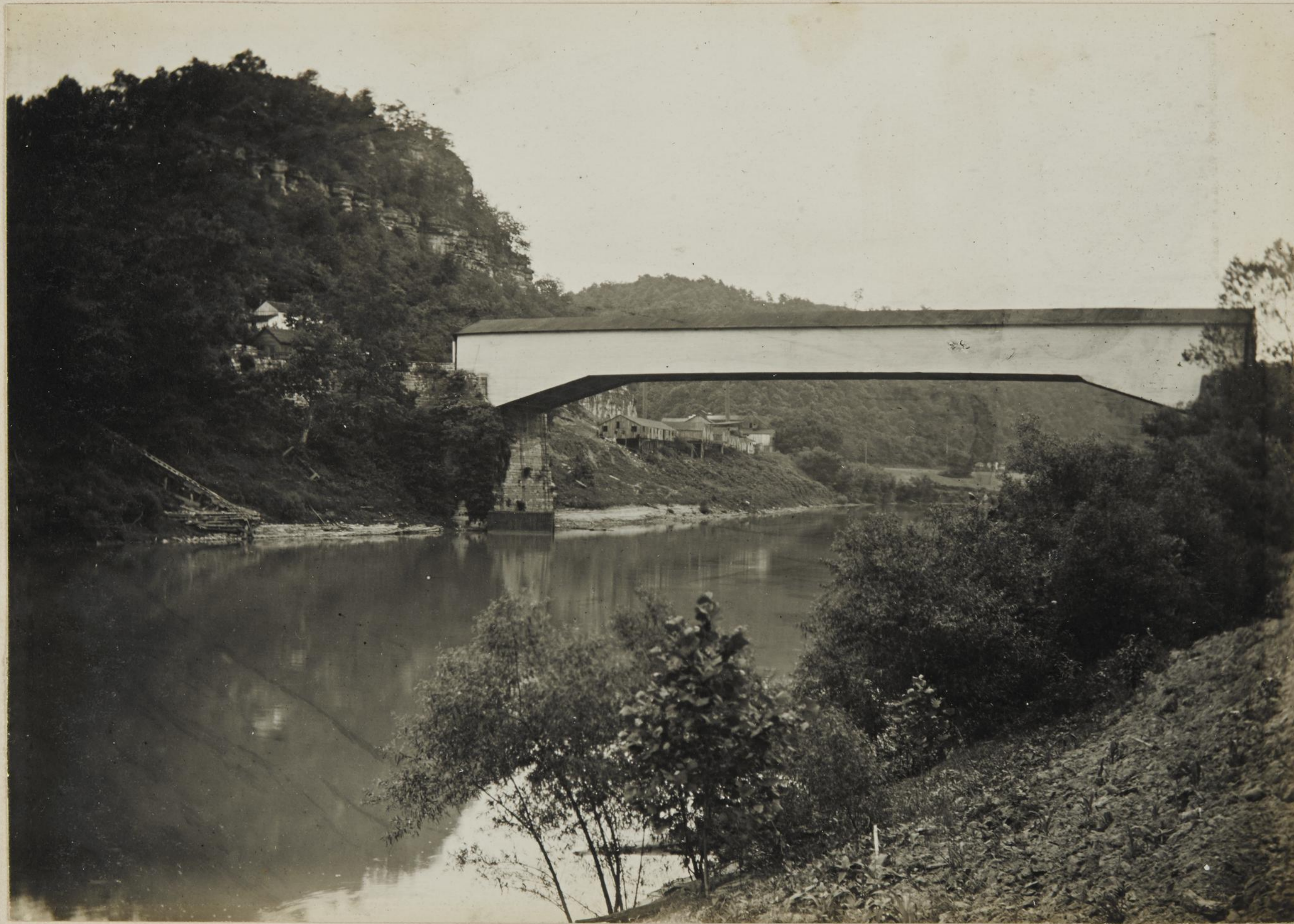
Single Span Wooden Bridge over Kentucky River - 1908. - Camp Nelson - Built in - 1838.
