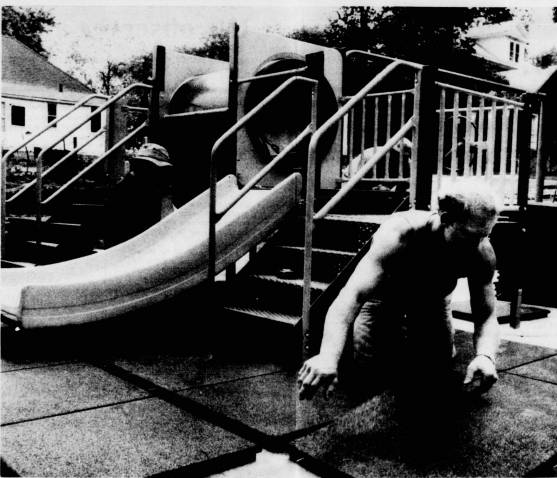
Dean Shepard of Hewitt Construction Company places rubber tiles over the concrete at the playground of the Kinder-Care Learning Center. The center, UK's first full-time, full-service day care, is scheduled to open in early August.
