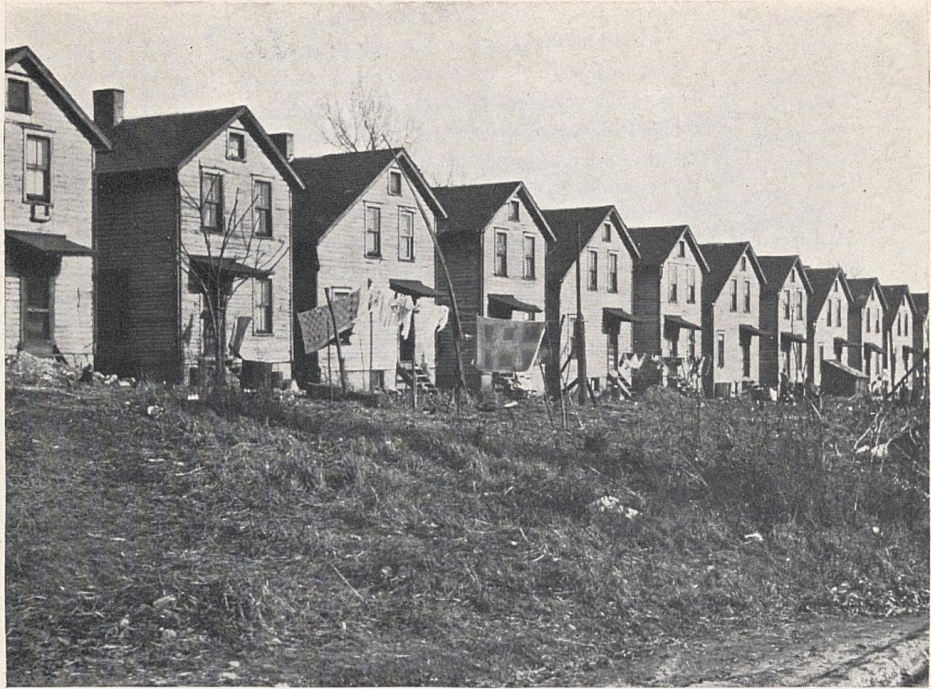
Before . . . Six out of seven of these Griffith Street shacks in Youngstown, Ohio, had no private toilets or bathing facilities. Three out of four were substandard.
