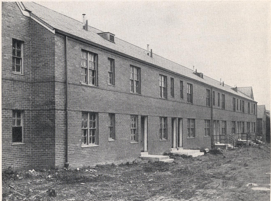
After . . . The Westlake Project, photographed from the same spot as above. Every home has a modern sanitary bathroom. Construction is fire-resistant throughout.
