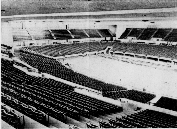
MEMORIAL COLISEUM, shown above, is finally nearing completion. The basketball floor was put down soon after this picture was taken and only the finishing touches now are left before the $4,000,000 structure will be opened for use by the University. This view toward the north end of the coliseum away from the main entrance, which is to the right. In the foreground are the individual seats. All other seats will be bleacher-type. It was announced last week that graduation services for the Class of 1950 will be held in Memorial Coliseum. The arena was started in March, 1947, and will be dedicated next month.
