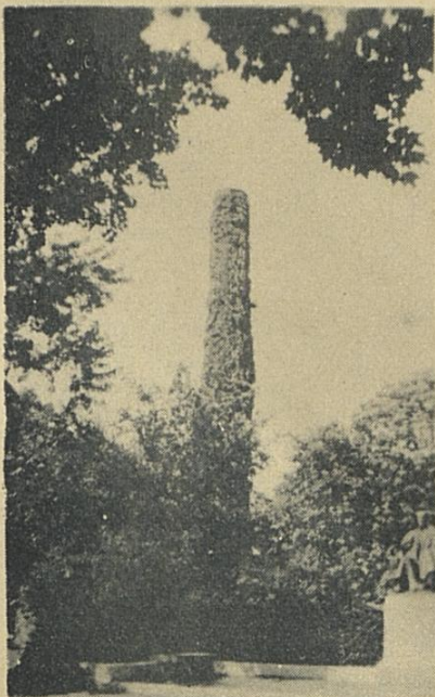
27 BELOW—OLD HEATING PLANT SMOKESTACK
