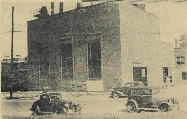
61 LEFT—NEW CENTRAL HEATING PLANT ON SOUTH UPPER
