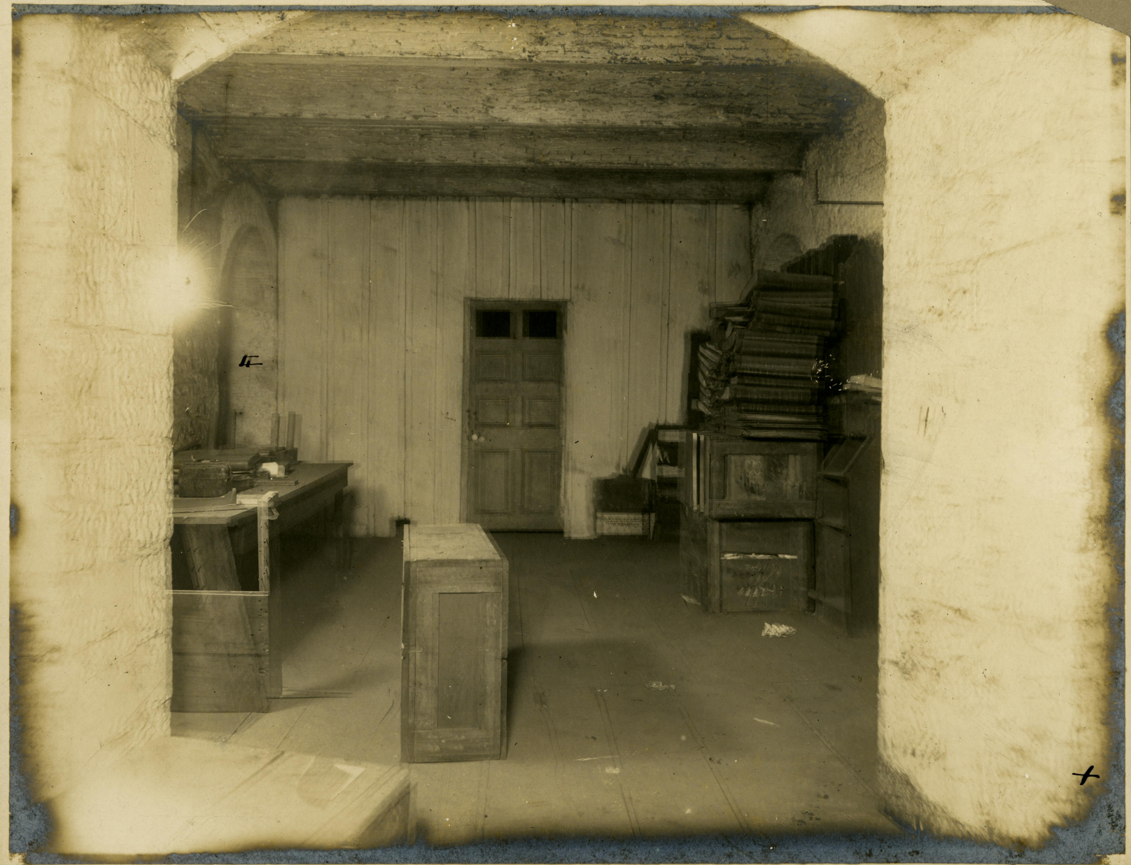
First basement room at bottom of steps and to right of them, coming down + shows bottom of steps - H shows entrance to 2 nd room leading to boiler stop - yellow note
