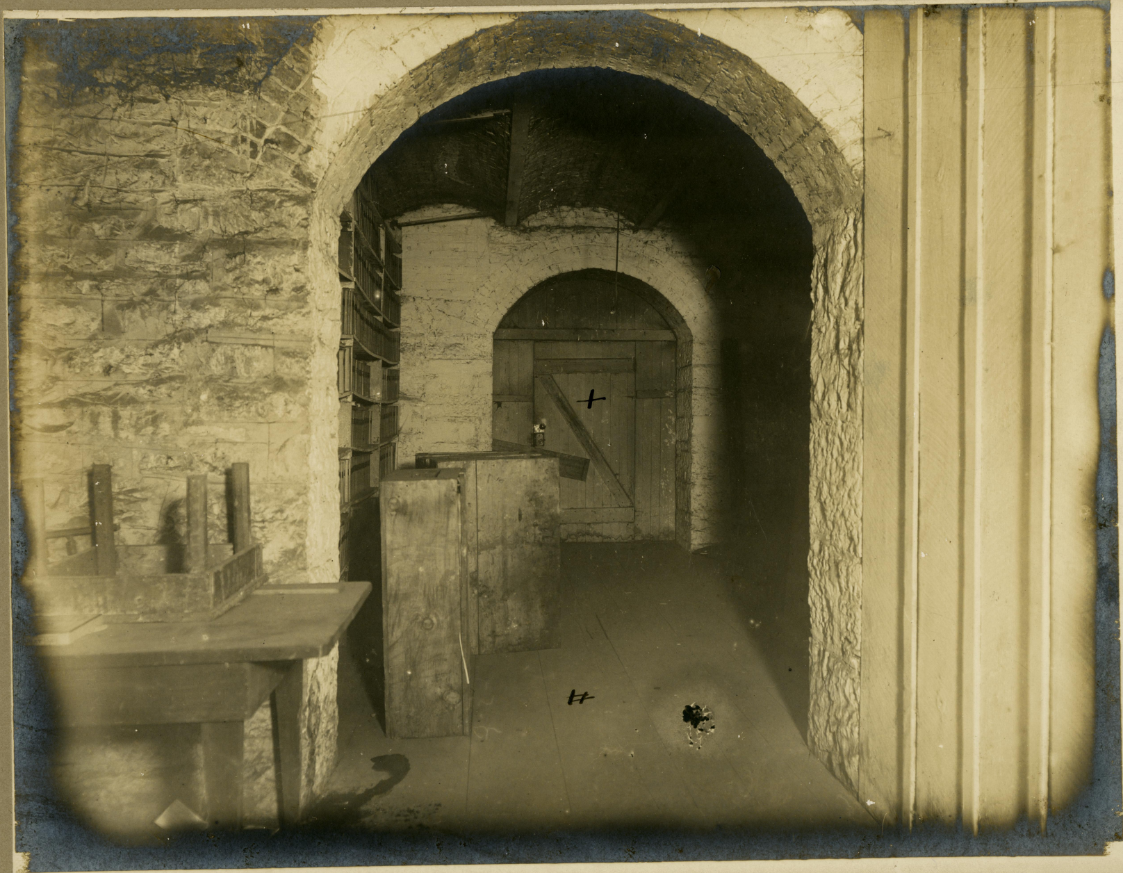
# shows 2 nd basement room, gallery, vault, + stairs door entering barby staf room of building and through which gallery ran =
