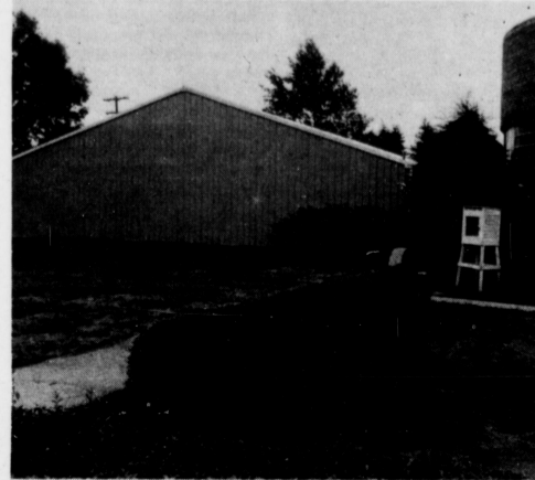
This unimpressive structure next to the Wenner-Gren building has—despite its appearance—an impressive function. Under construction inside is a 50-foot centrifuge which may help make extended space flights more comfortable for astronauts.
