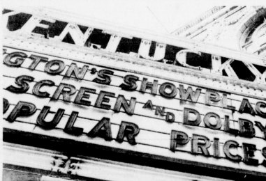
The Kentucky Theater, which suffered fire damage in October, is still closed.
