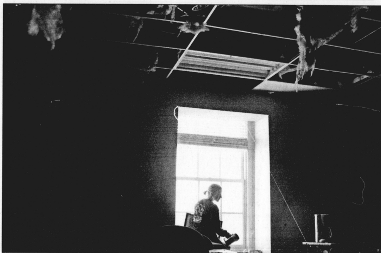
Above: Crystal Bruno sits in the window and surveys the damage done to Jennings Hall, a classroom building at Union University. Jennings Hall lost portions of its roof during the storm on Tuesday, which led to flooding later in the night. Top Right: A car sits overturned as a result of the tornado that touched down at Union University on Tuesday night. Classes at Union are not expected to resume until after Feb. 18.
