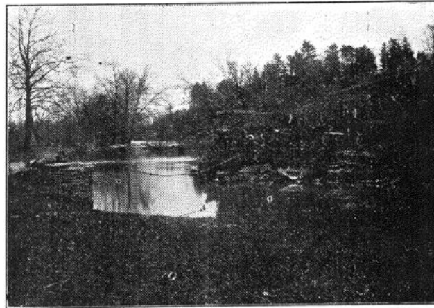
SHOWING THE OLD ABUTMENT.
