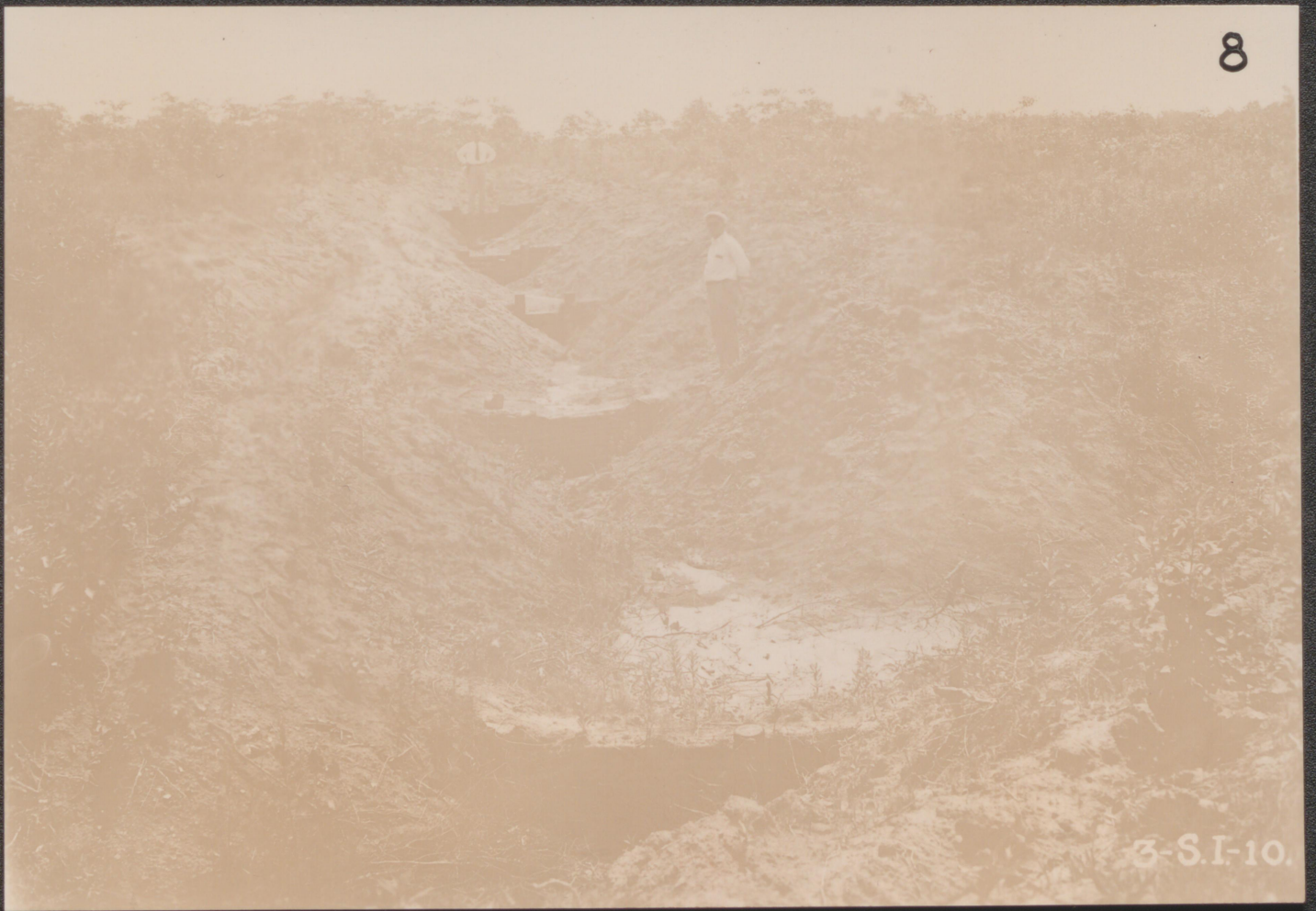
Series of dams to stop erosion in one small gully.
