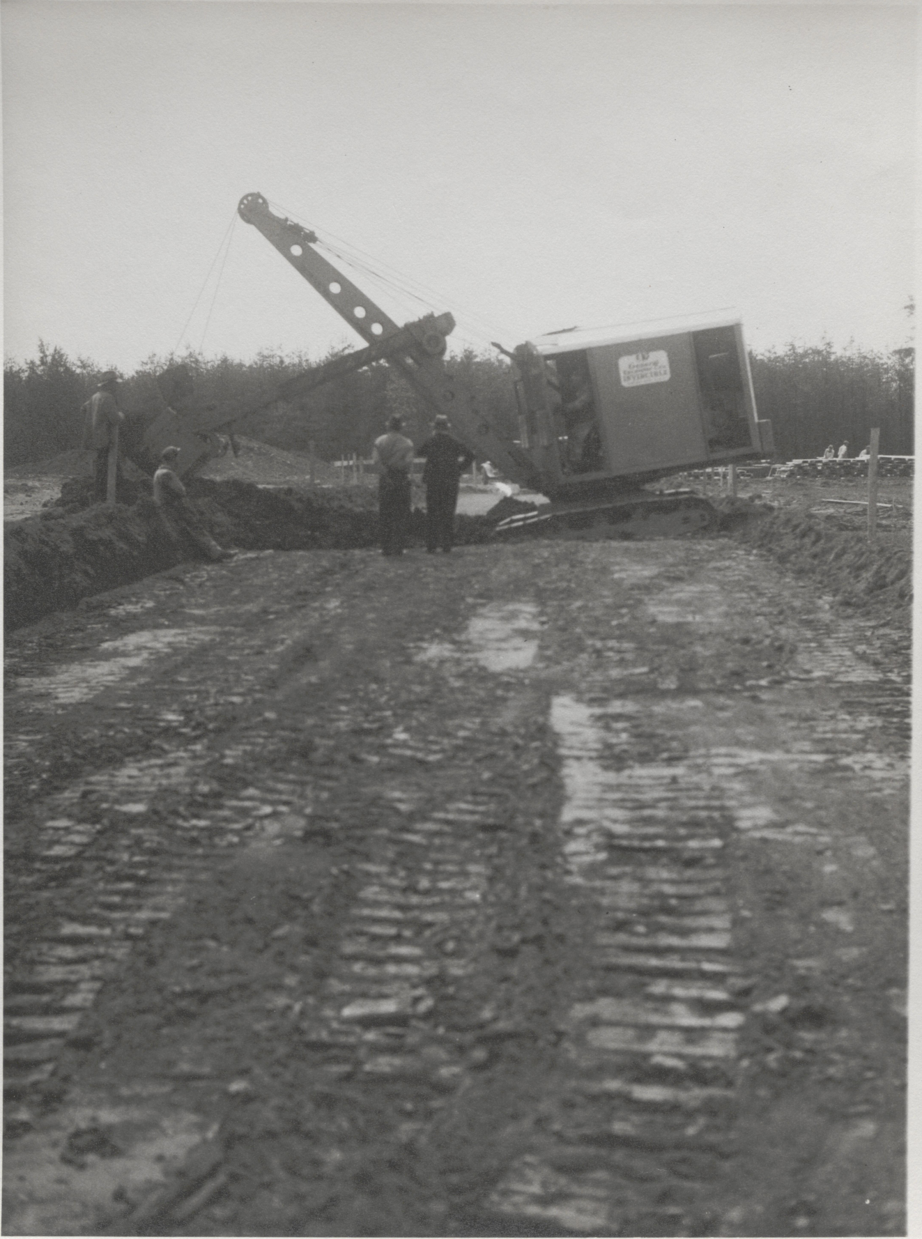
2. MACHINE EXCAVATION UNDERWAY
