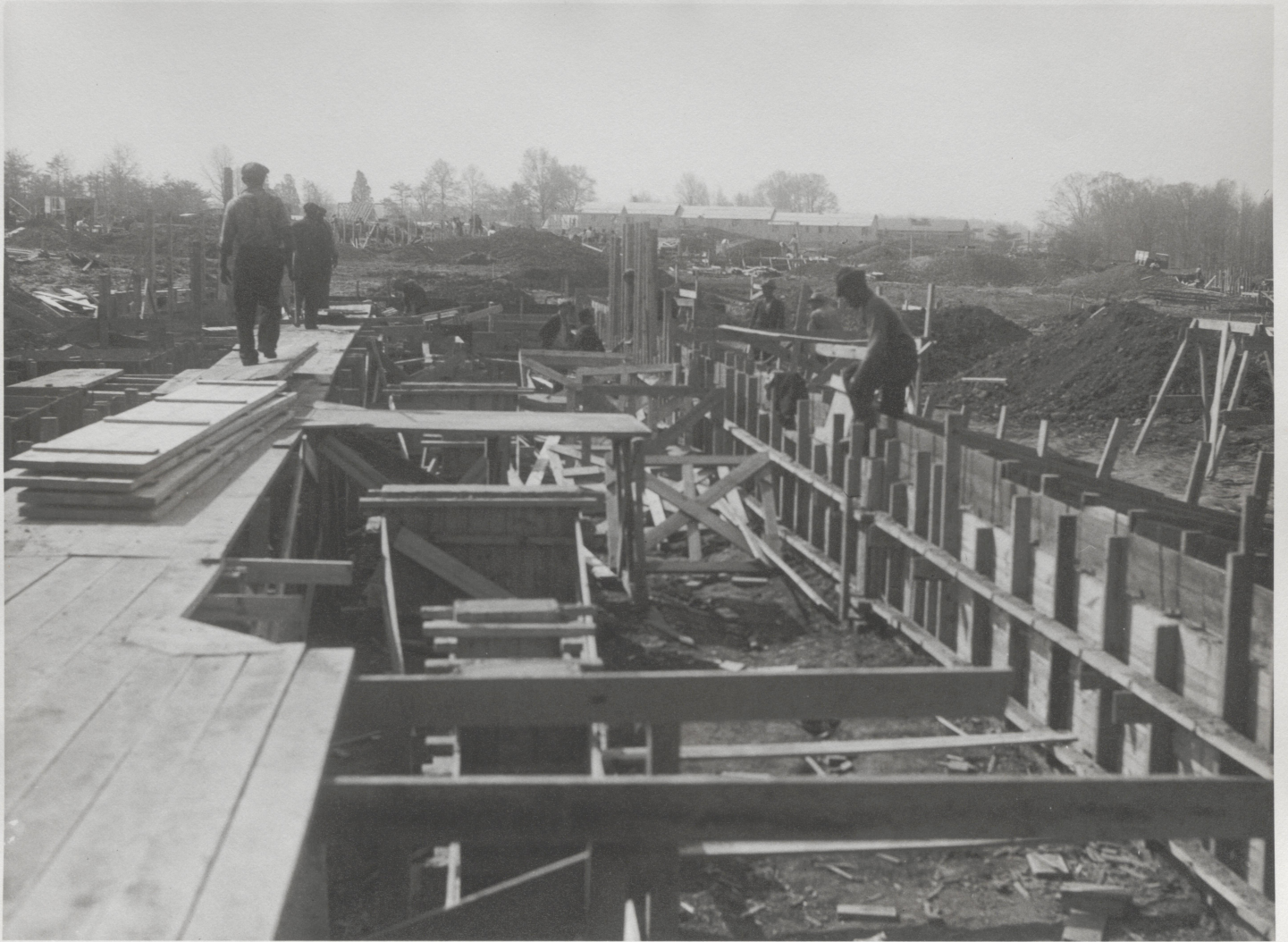
9. WALL FORMS POURED
