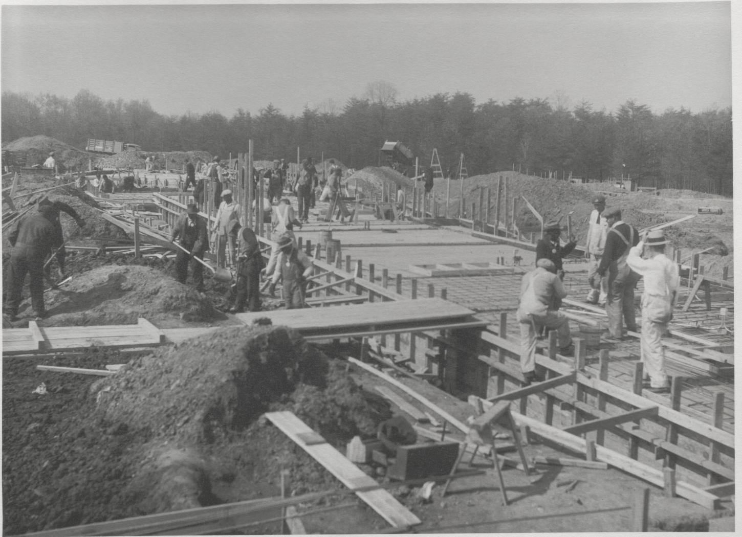
14. FRAMING - STUDDING ERECTED
