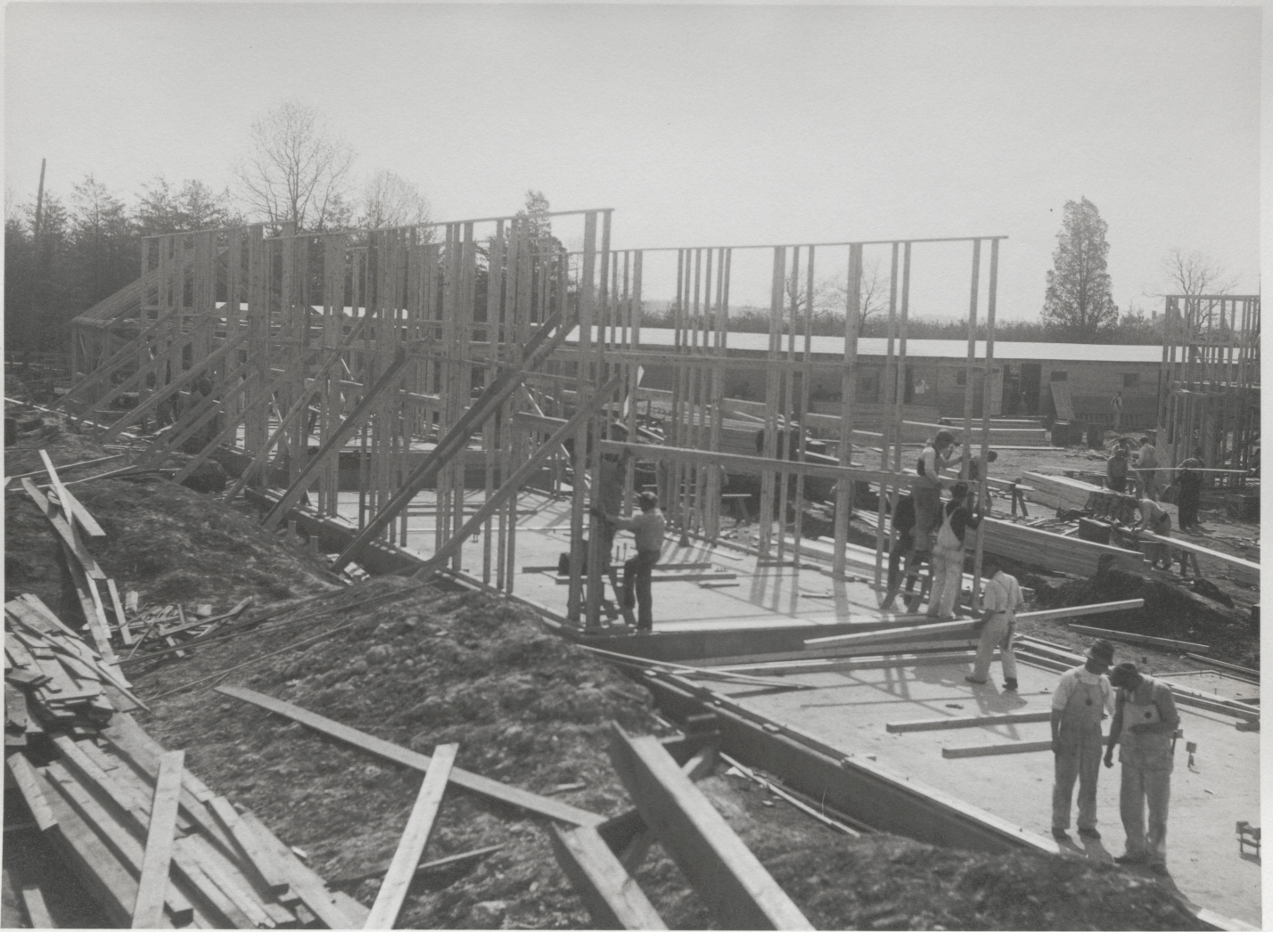
15. FRAMING - FLOOR JOISTS, SHEATHING STARTED, PARTITIONS STARTED
