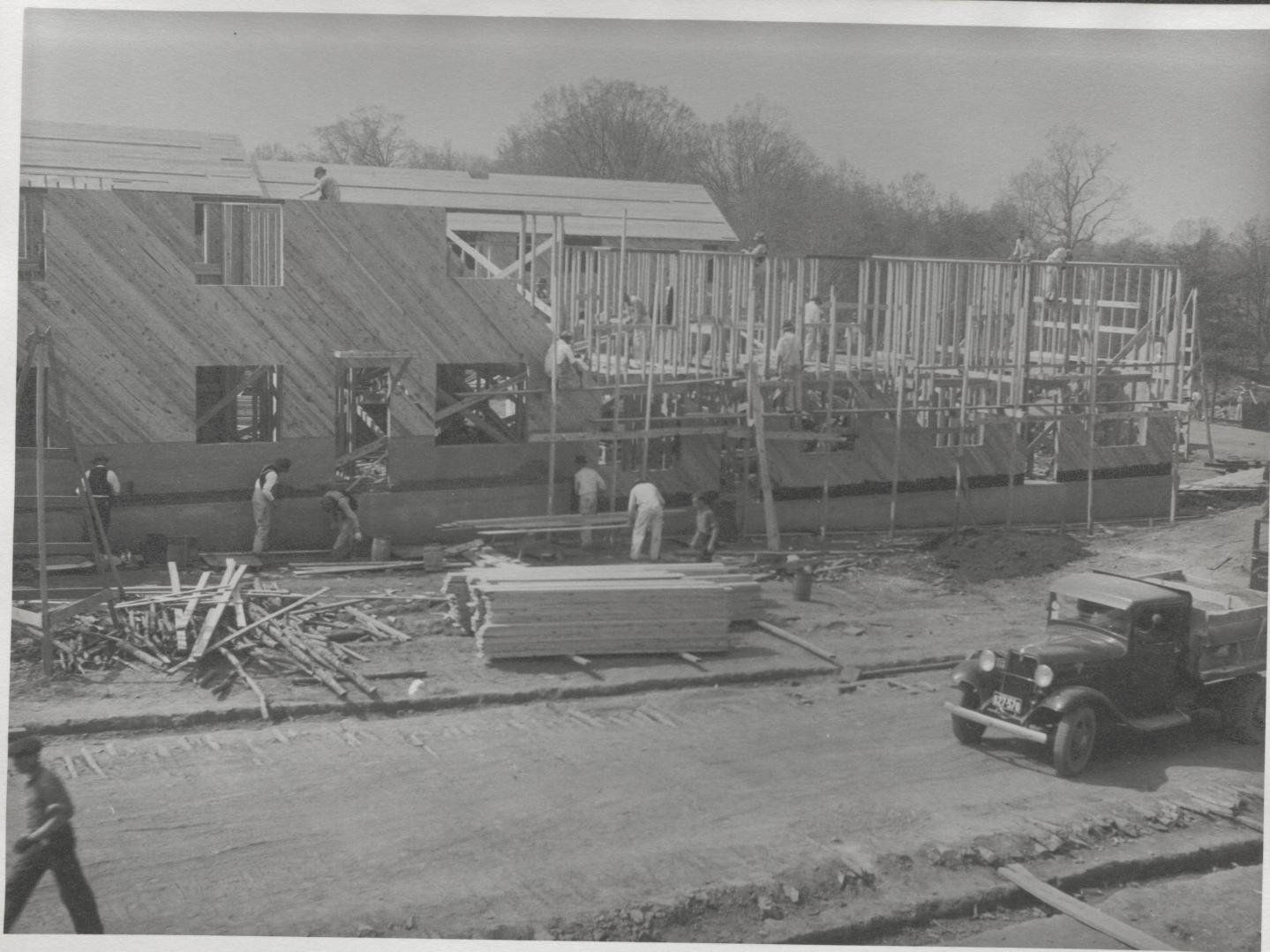
16. FRAMING - BRICKWORK JUST BEGINNING
