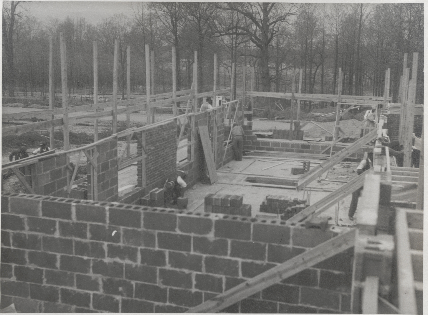
24. CINDER BLOCK - INTERIOR VIEW SHOWING INTERIOR WALLS
