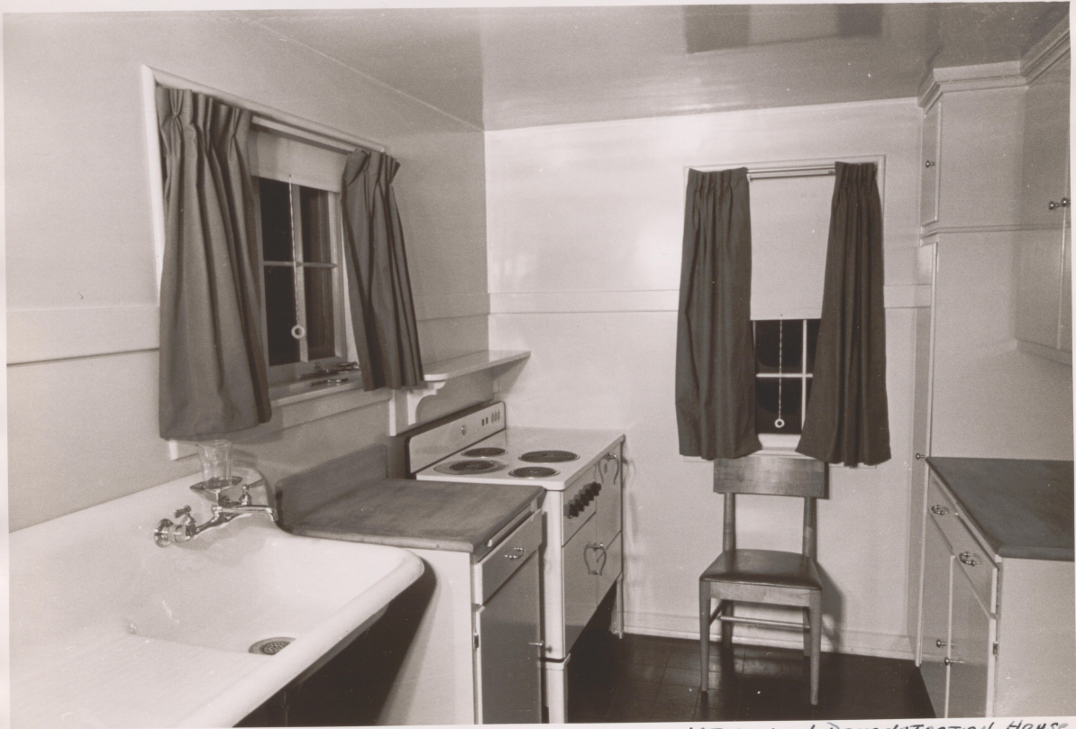
KITCHEN IN DEMONSTRATION HOUSE Type F-12
