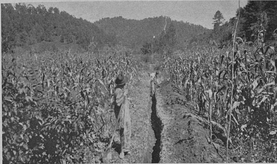
The productive capacity of farm land is often more than doubled by proper drainage. The tile drainage on this Knox County farm was possible only after a stream bed had been cleared and deepened.
