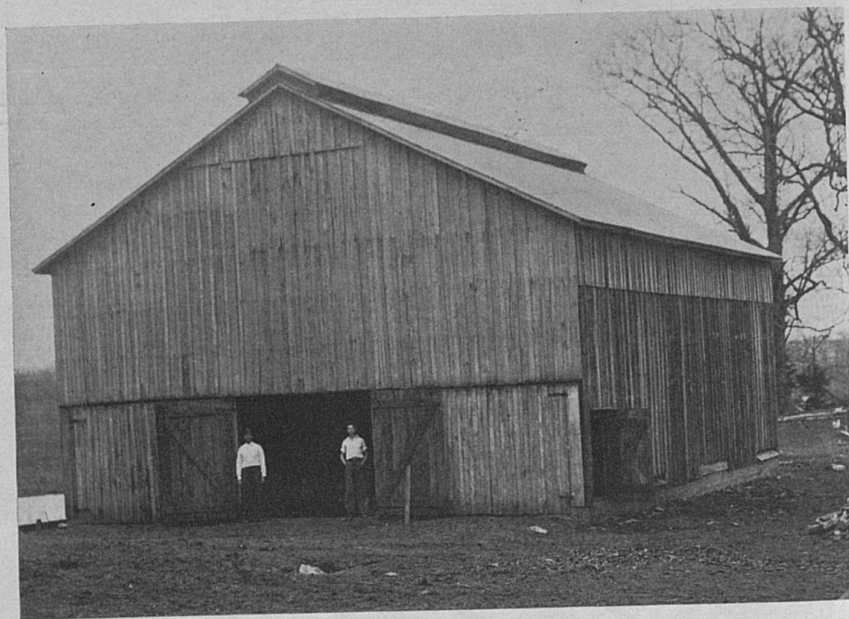
Eight modern, ventilated tobacco barns resulted from the construction of this tobacco barn in Caldwell County. Note the ridge ventilator.
