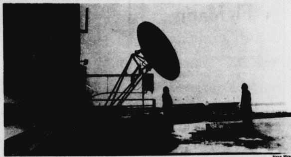
RCA engineer Joe Moore, left, and Ralph Brown of the UK Medical Center examine an antenna used to send and receive microwave transmissions. The antenna is perched atop the Medical Center.
