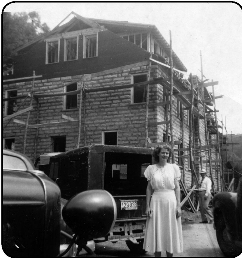
This photo shows construction of the Margaret Voorhies Haggin Quarters for Nurses.
