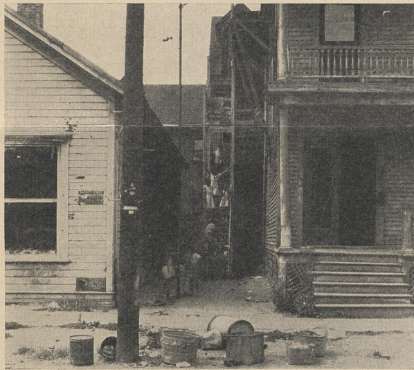
Six families (11 adults and 10 children) lived in this Syracuse tenement now replaced by the Eastern project. They paid from $12 to $17 monthly rent, and were without either private baths or private indoor flush toilets. The wooden fire escape is the only exit for those living on the third floor.
