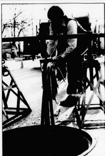
Cable connection Donny Smith, an employee of the UK Physical Plant Division, guides cable into a manhole on Hilltop Avenue yesterday.
