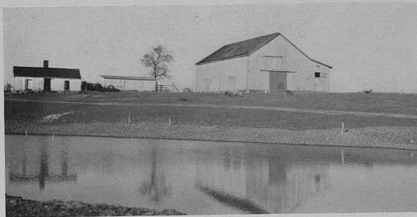
FIGURE 6. A farm reservoir protected from silting by permanent sod. Note electric fence to exclude livestock.
