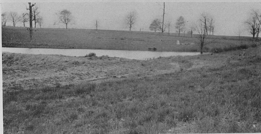
FIGURE 12. Farm reservoir with spillway at end of dam, protected from erosion by bluegrass sod.
