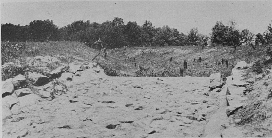
FIGURE 11. Upper portion of spillway protected from erosion by vegetation, lower portion by rubble masonry.
