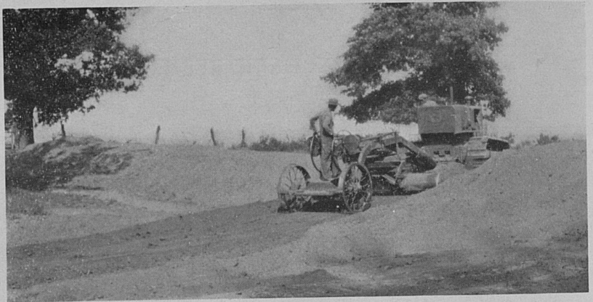
FIGURE 1. Crawler type tractor and two-wheeled terrace grader used for building farm reservoirs.
