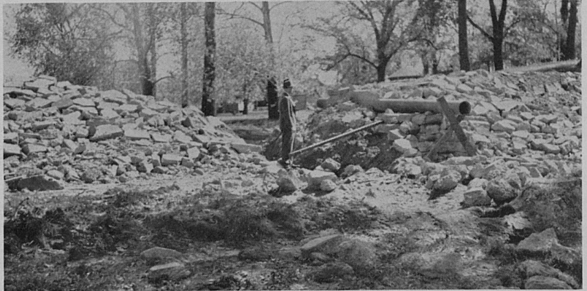
FIGURE 4. Break in an earth dam due to inadequate spillway.
