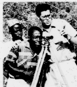
ROAD SURVEYING techniques are explained by Volunteer Eugene Schreiber to co-workers in Tanganyika. Schreiber, 21, is a civil engineering graduate of Purdue University.
