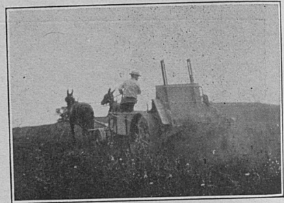
Twenty minutes are required for two men to load and spread a two-ton load of marl with a portable chute and a manure spreader.
