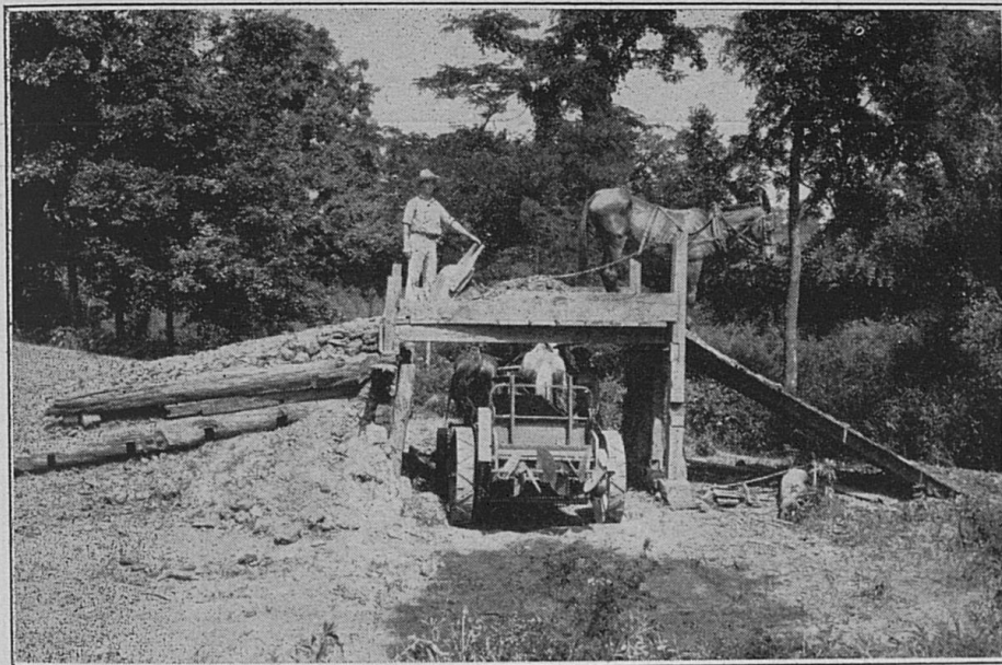
Trapdoor method of loading marl.
