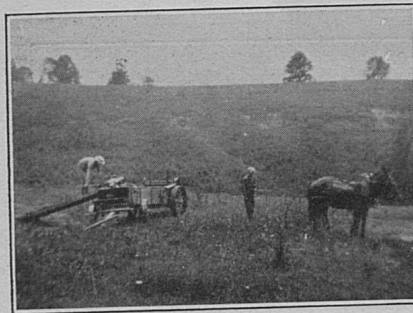
Twenty minutes are required for two men to load and spread a two-ton load of marl with a portable chute and a manure spreader.
