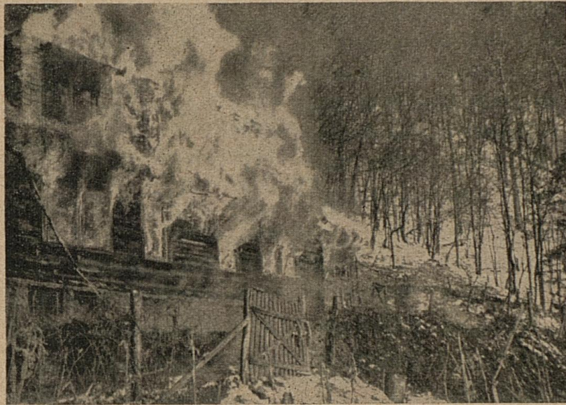
Fifteen Minutes After the Alarm. Water Now Played Entirely on Part of Building near the Safe.
