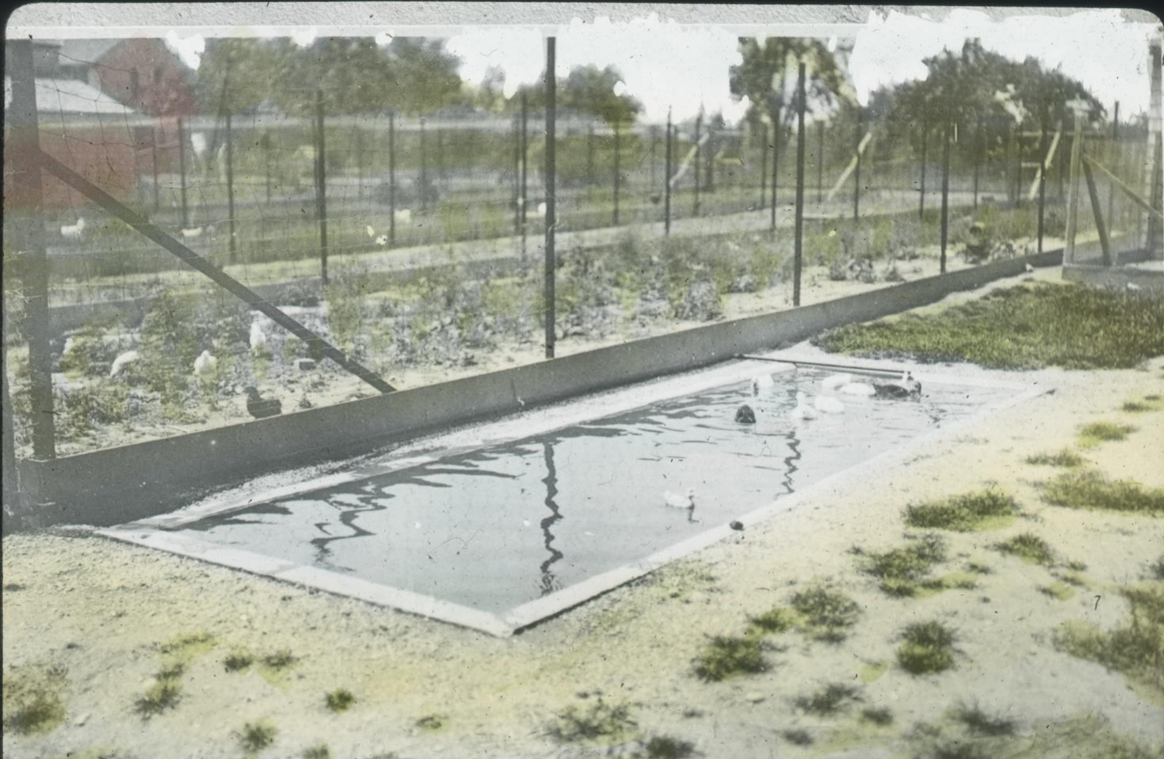
Concrete Swimming Tank for Poultry — No turtles or varmints to kill young ducks. Dimension 12'x6'x8"deep. Cost $11.22
