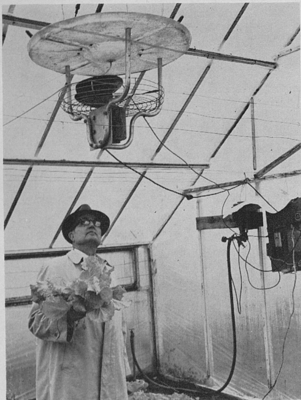
Horticulturist Emmert inspects equipment used to circulate heat and air and to keep the relative humidity constant in a plastic greenhouse. Note the baffle plate which deflects the forced air downward.
