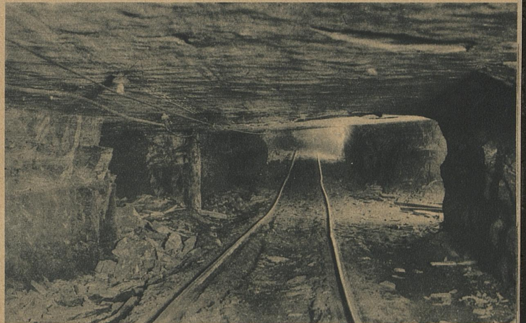
Entry way in a mine
