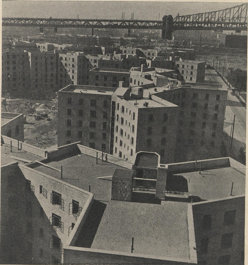
TYPICAL QUEENSBIDGE OFFSET Y-UNITS. Almost 2,500 American cities and towns are smaller than this complete community which spreads over 47 acres at the Long Island end of New York's great Queensborough Bridge. Some 11,400 people, liberated from the Nation's most congested slums, will learn to live in fresh air and sunlight, will see garden walks, trees, and green grass through well-spaced apartment windows. Wives used to tenement hardships will discover modern bathrooms, electric refrigerators, gas stoves, and generous closets. Here slum children can romp safely on Queensbridge playgrounds. (Photo by McLaughlin Air Service.)
