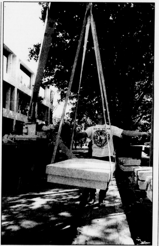
HAVE A SEAT Ray Lockwood, of Baker Concrete, prepares the sandstone caps that will be set in concrete today in front of White Hall Classroom Building. The caps will finish the seating wall that was started earlier this semester.
