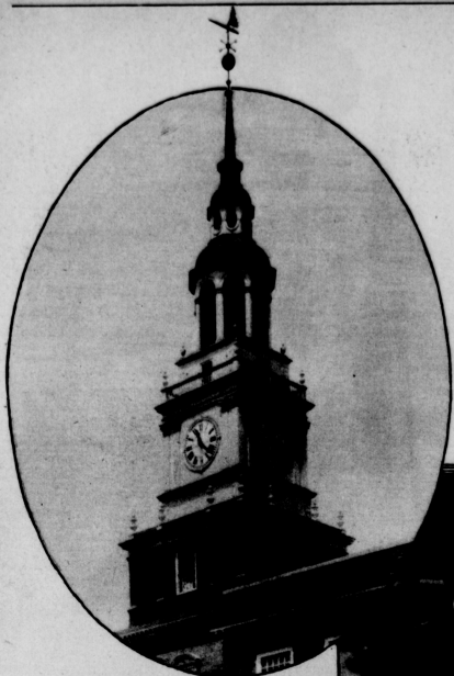
A New Tower Rises on Dartmouth Campus —It tops the new million-dollar Baker Memorial Library—a beautiful example of the simpler type of Colonial Georgian architecture. The new library has accommodations for 550,000 books and its reading rooms can seat 1,000 students. It is the gift of George F. Baker. (The Dartmouth)
