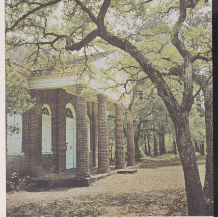
St. James Santee Church was built in 1768 from brick shipped from England.
