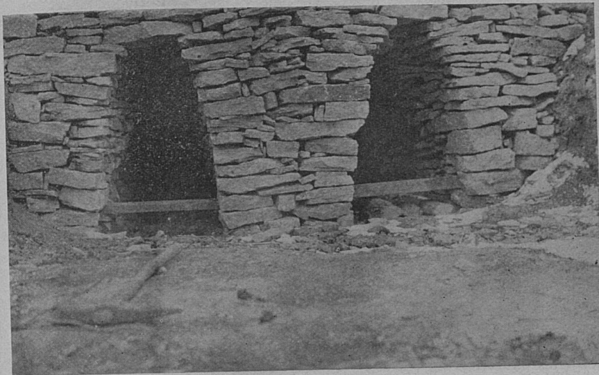
Limekiln built in Breckenridge County under the direction of Agent Joe Nageotte and Earl G. Welch from the College of Agriculture.
