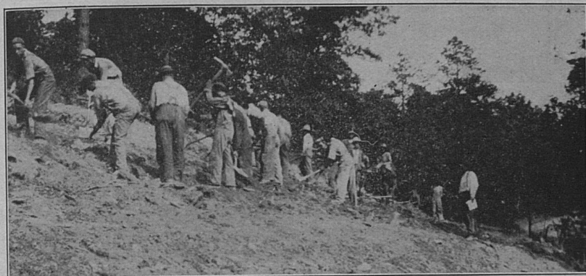
Lee County road working day.
