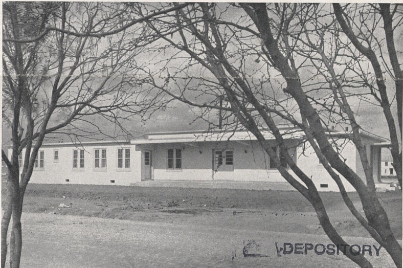
Stucco-finish administration building at Kinney Place, where 134 families will pay $13.25 a month for shelter and utilities.
