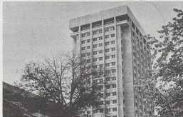
PATTERSON OFFICE TOWER —The 19-story tower houses more than 1,000 faculty members, primarily in Arts and Sciences, Library Science, Social Professions, Student Affairs, and the Patterson School of Diplomacy. The top floor has well-appointed meeting and conference rooms, lounges, and an observation area. The WHITE HALL CLASSROOM BUILDING —adjoining the Patterson Tower with both underground and above ground walkways, features large modern classrooms which accommodate nearly 4,000 students. It is one of the largest structures of its kind in the nation.
