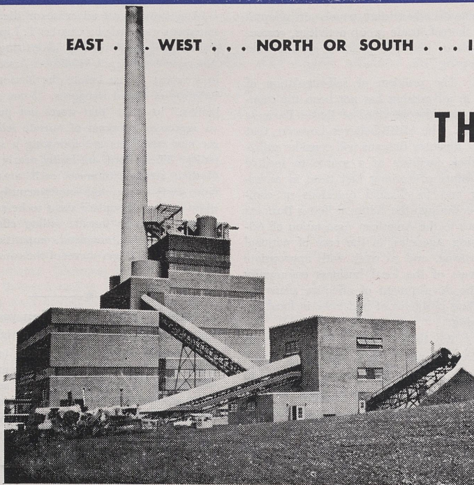
E. W. BROWN GENERATING STATION on Herrington Lake near Dix Dam
