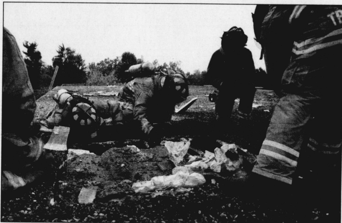
Lt. Tim May (black helmet) leads a crew of trainees on the roof of the former Pi Kappa Alpha fraternity house in a routine ventilation process.
