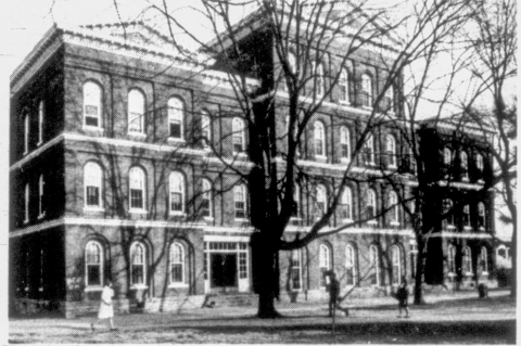
White Hall, top, and Patterson House were razed this spring to make way for a new classroom-office complex. They were two of the oldest buildings on the campus and represented much of the University's 102-year history. Their passing also represents many of the changes sweeping the campus.
