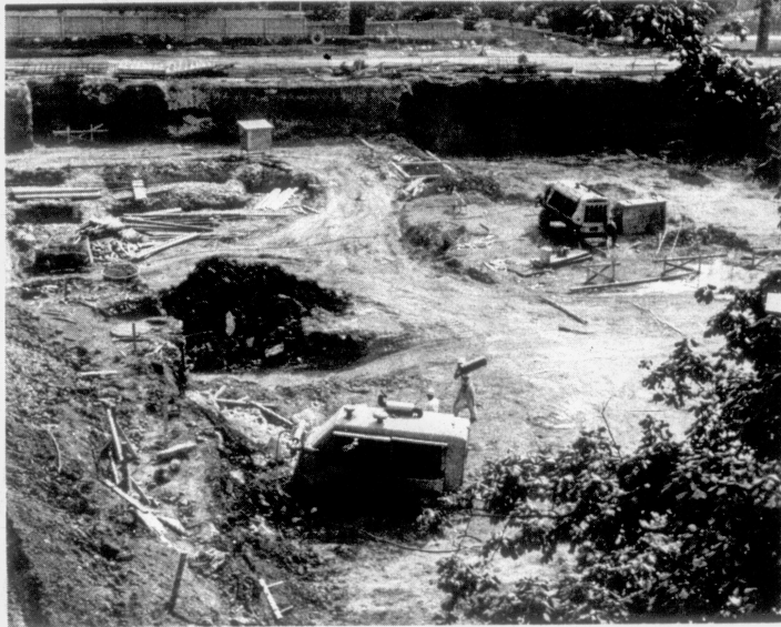
Construction Got Underway This Spring On A New Office-Classroom Complex
