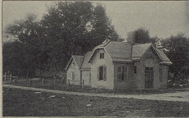
DAIRY BUILDING—EXPERIMENT STATION FARM.
