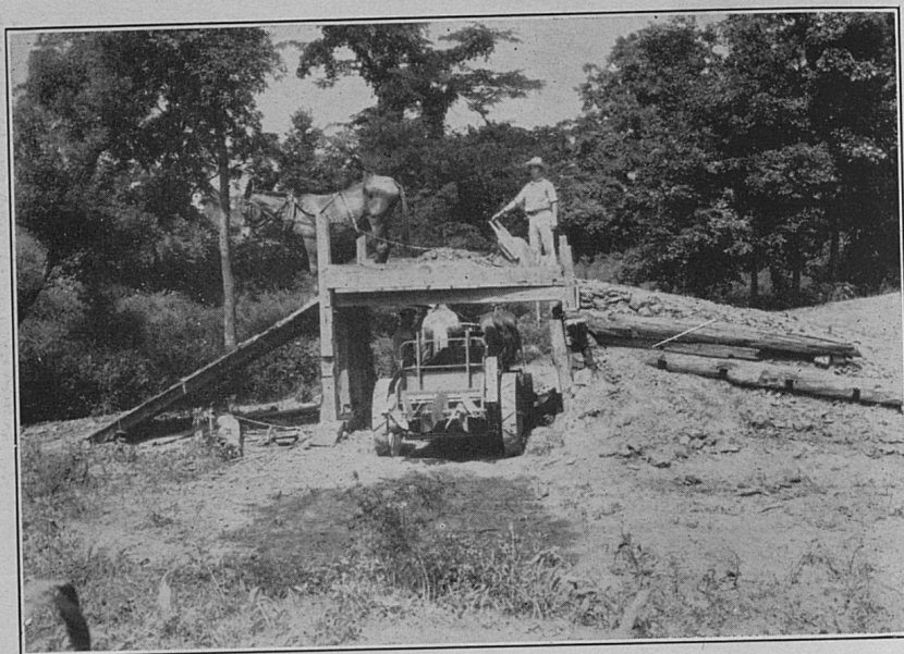
Loading marl with trap-door loader.
