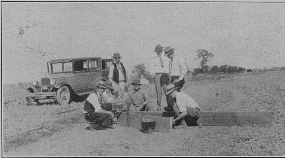
Building a terracing drag.
