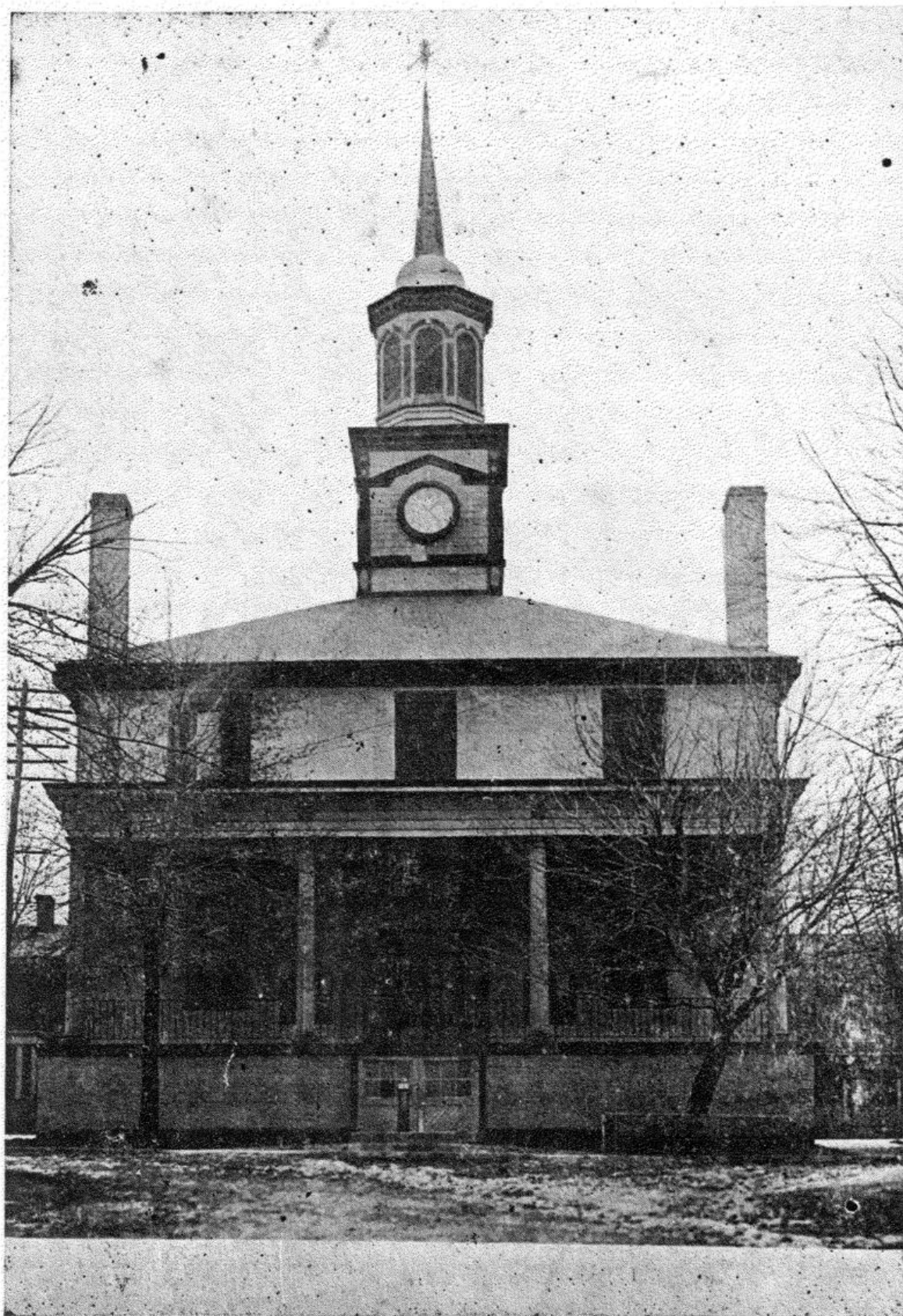
COURT HOUSE, FLEMINGSBURG, KY.
