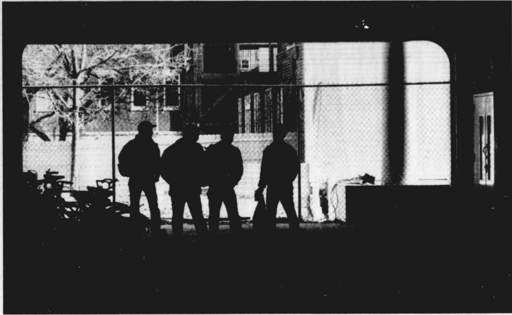
Construction workers began excavating areas on campus as part of plans for a new civil engineering building. Unauthorized people are not allowed near the excavation site. For related story on campus construction, see Page 3.
