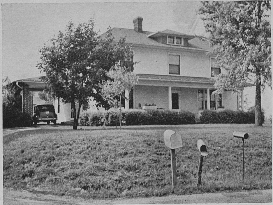
Terraces are difficult to build and maintain and should be omitted wherever possible.
