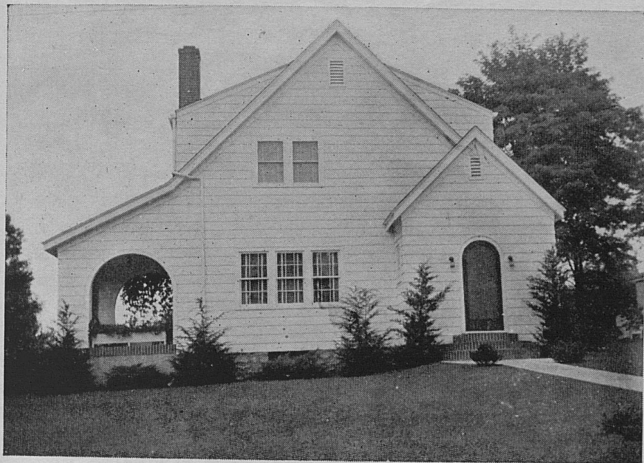
A new lawn that was well graded before it was seeded. Notice how it is graded up to the walk and away from the house. This means the water runs from the foundation of the house and from the walk.
