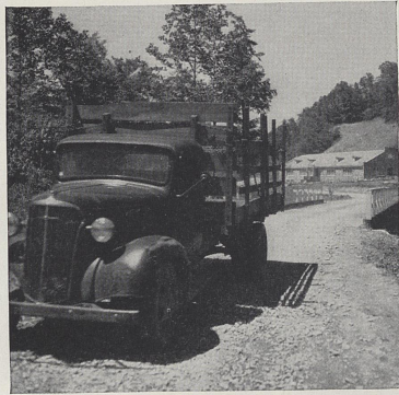
After WPA road work is done, the farmer can speed to town at will. This work includes straightening and broadening the road, reducing steep grades, providing adequate drainage, building culverts and bridges, and surfacing the road (with local materials if possible).
