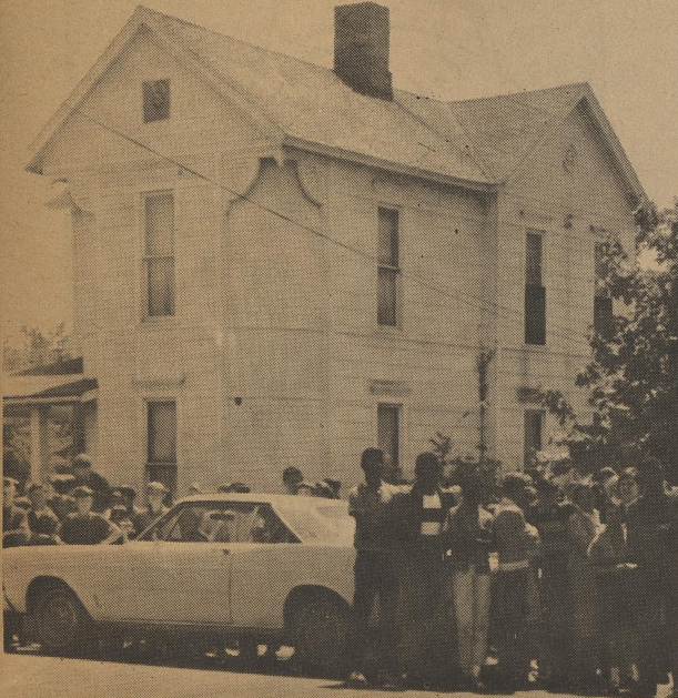
Lowell Hobby and Gid S. Pool purchased the CALDWELL COUNTY TIMES on June 11th, 1966. The space was limited, with a building a little more than 17-feet wide. The company purchased the old historical house (in photo) at public auction July 1, 1967. It was quickly demolished and a new building was started. The site is located just 4-blocks from the prior location which was on "court house square".
